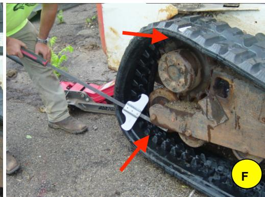
By using the Hammerhead the span of the tool allows for easier and more precise placement of the cogs on the tracks. This wider base tool prevents damage to the new track because three points are moving the track with a span of 10" instead of one point that is 1" wide. Once the drive has been set over the drive gear (C,D,E), apply pressure to the track to skid it over the lower idler (F).
